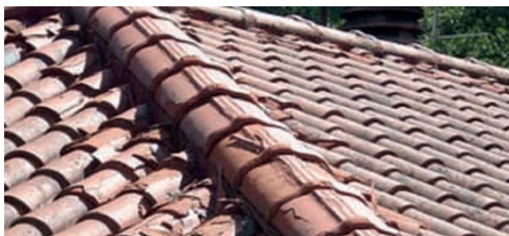
Example of a poorly ventilated roof
